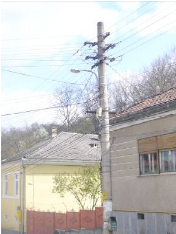
Picture: street lighting in Dej, RO:
